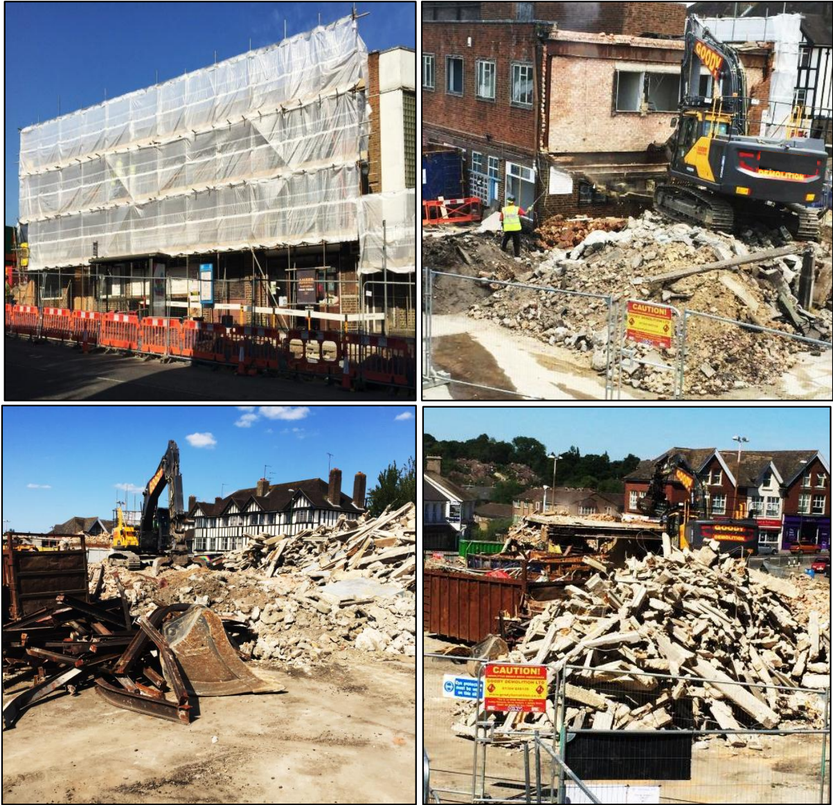
Figure 7.1: Sample of demolition works at the demolition site.
